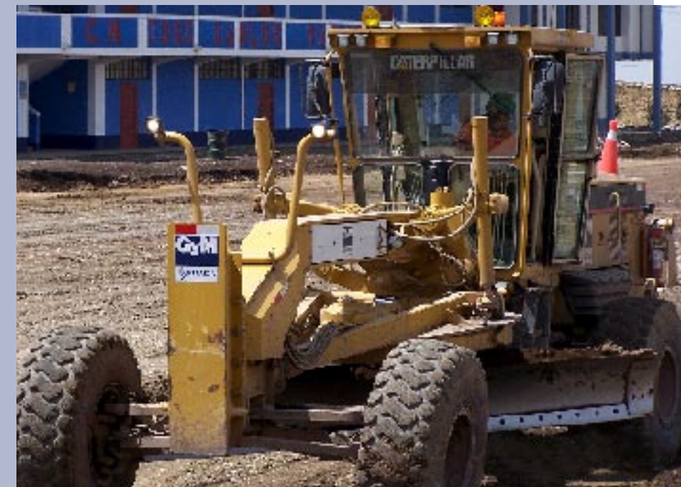
160H GRADER CARRYING OUT THE FINAL TRIM ON THE NEW SPORTS FIELD
