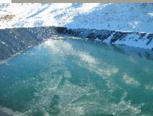
CONSTRUCTION OF ROCKY GULLY RESERVOIR
